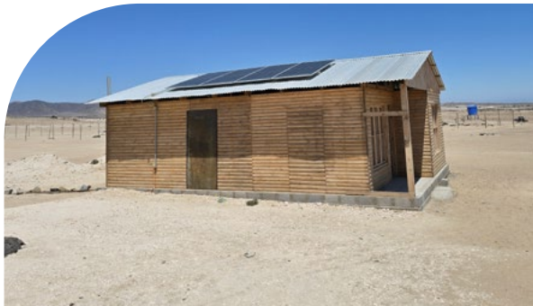
Rooftop Solar Kit donated to Wentu Lafquen and Emma Piñontes Indigenous Community house - Calderaza (Chile), NextEnergy 3
